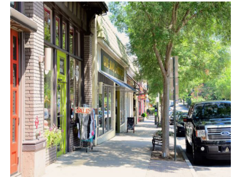
Single Story Shopfront
